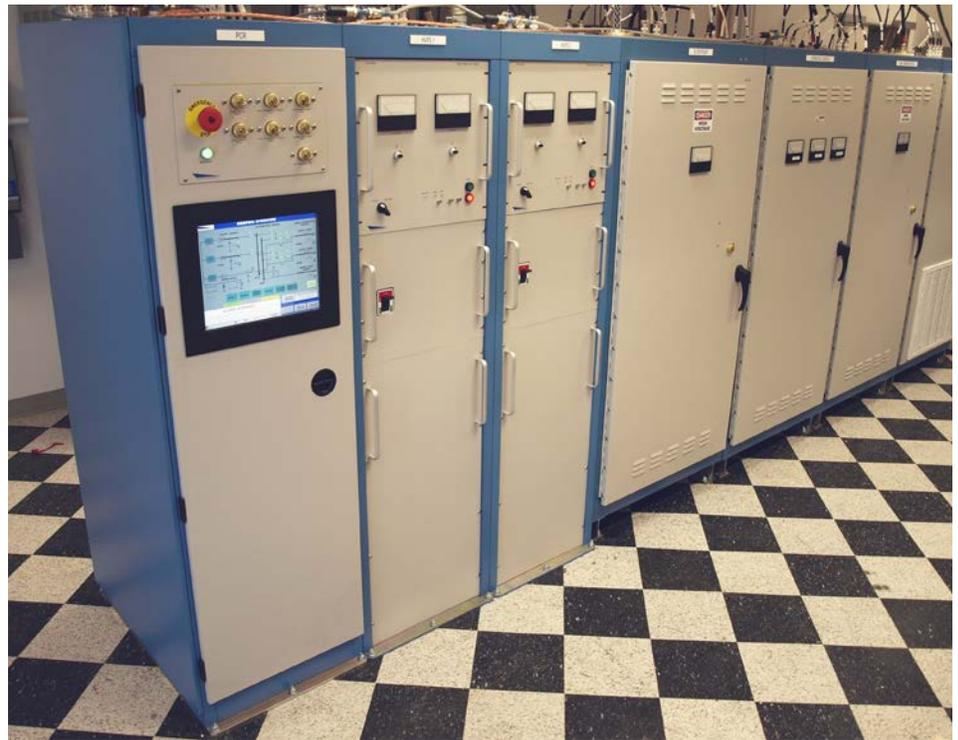
**Power Feed Equipment for the MVDC Conversion and Transmission System.** This system is shore-located and is housed in two 20-foot ISO containers and powered by two 200 kV high voltage power supplies run in parallel.
