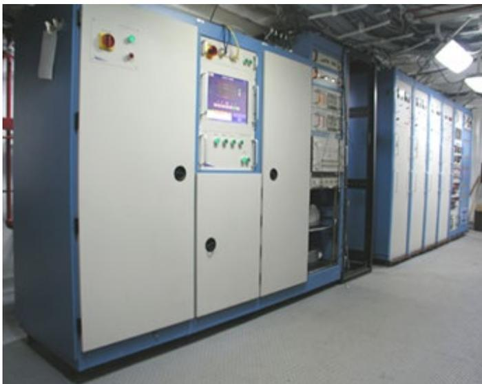
Figure 2. Cobra Judy X-band DC power supplies and controls installed on-board the USNS Observation Island.
