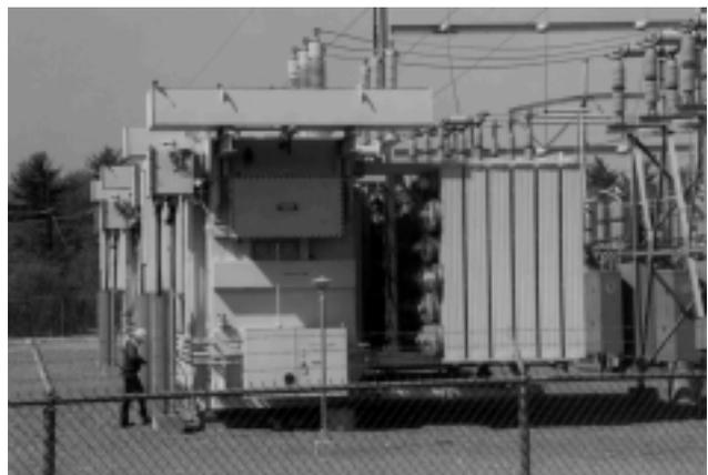
*Figure 2: 115kV to 13.8kV AC Transformer*
