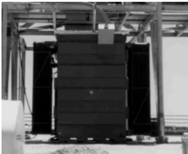
Figure 4: 2 MW Transformer
