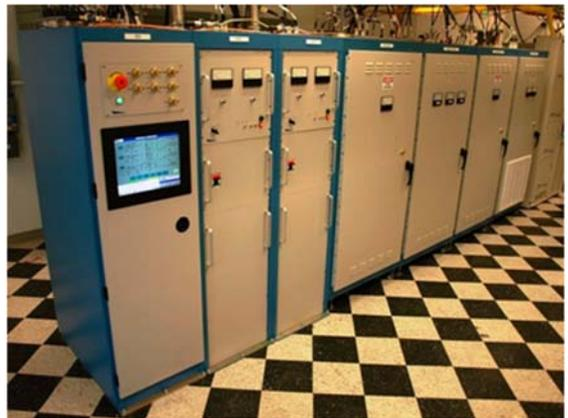
Figure 2. Installed Shore Power Feed Equipment.
