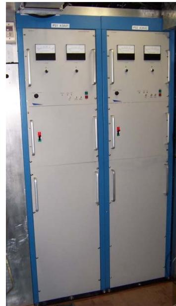
Figure 7. DTI COTS 200 kW, 20 kV power supplies.
